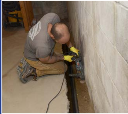
2. Drill holes in footing.
