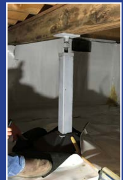
7a. Alternative on-grade installation
