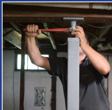
6. Fully tighten stabilizer
