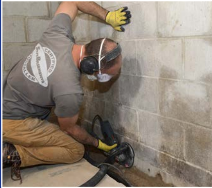
1. Prepare wall for Carbon Fiber.
