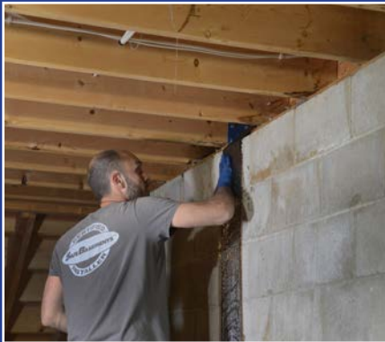
4. Install Carbon Fiber on wall (from the top down).
