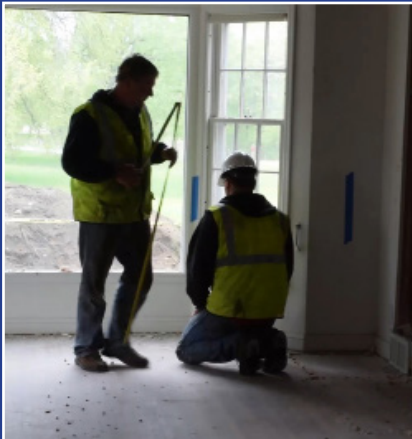
5. Measurements are made and the foundation is lifted to level.
