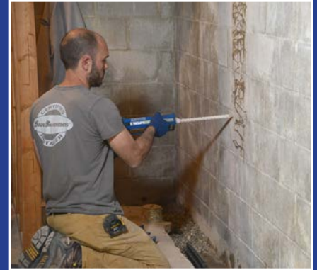
3. Add epoxy to prepped area on wall.
