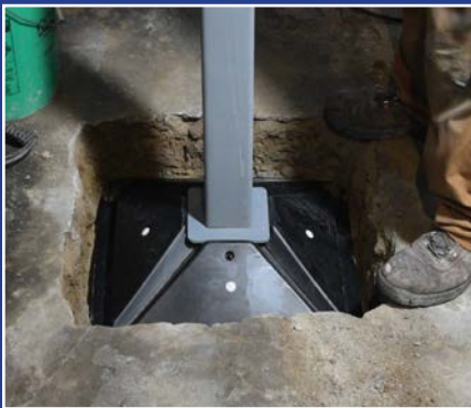
3. Place and secure stabilizer on the LightFoot base
