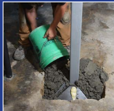
7. Replace and finish concrete where necessary
