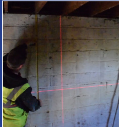
6. Measurements are confirmed again after. Cylinders are removed and backfill can begin.
