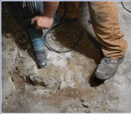
1. Prepare soil for footing placement
