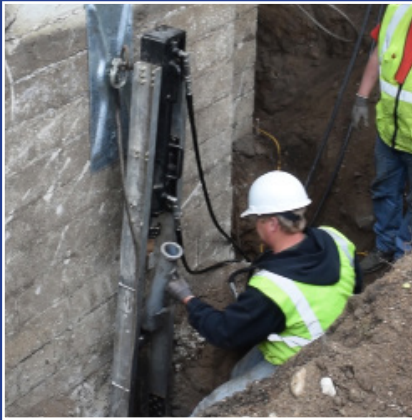
3. A hydraulic ram is used to push the pier to bedrock or load bearing strata.
