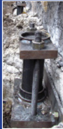
3. A hydraulic ram is used to push the pier to bedrock or load bearing strata.
