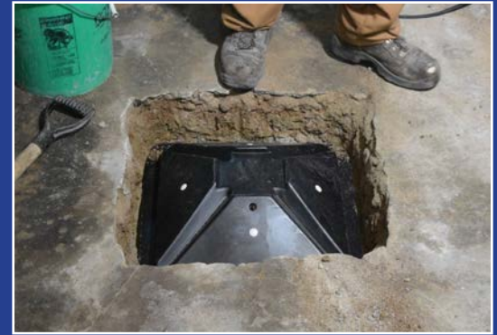
2. Place LightFoot into prepared space
