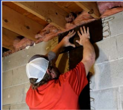
5. Install second Carbon Fiber strap horizontally (at top).
