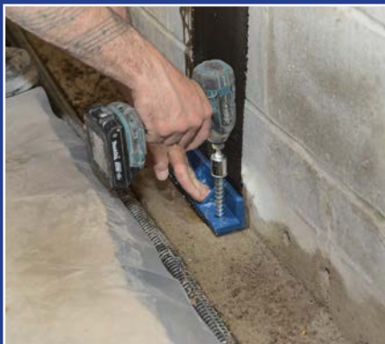
7. Add & secure base bracket to footing or floor.
