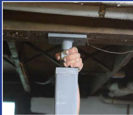
3. Place and secure stabilizer on the LightFoot base
