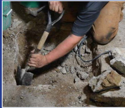
1. Prepare soil for footing placement
