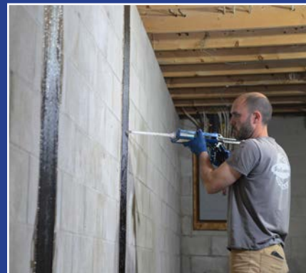
8. Add epoxy to Carbon Fiber.
